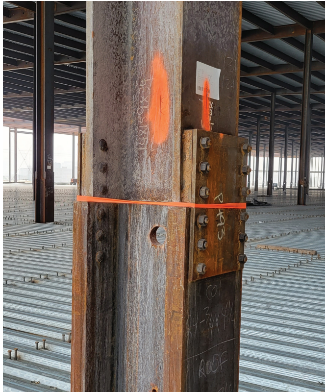
Fig. 1. Bolted column splice example.
