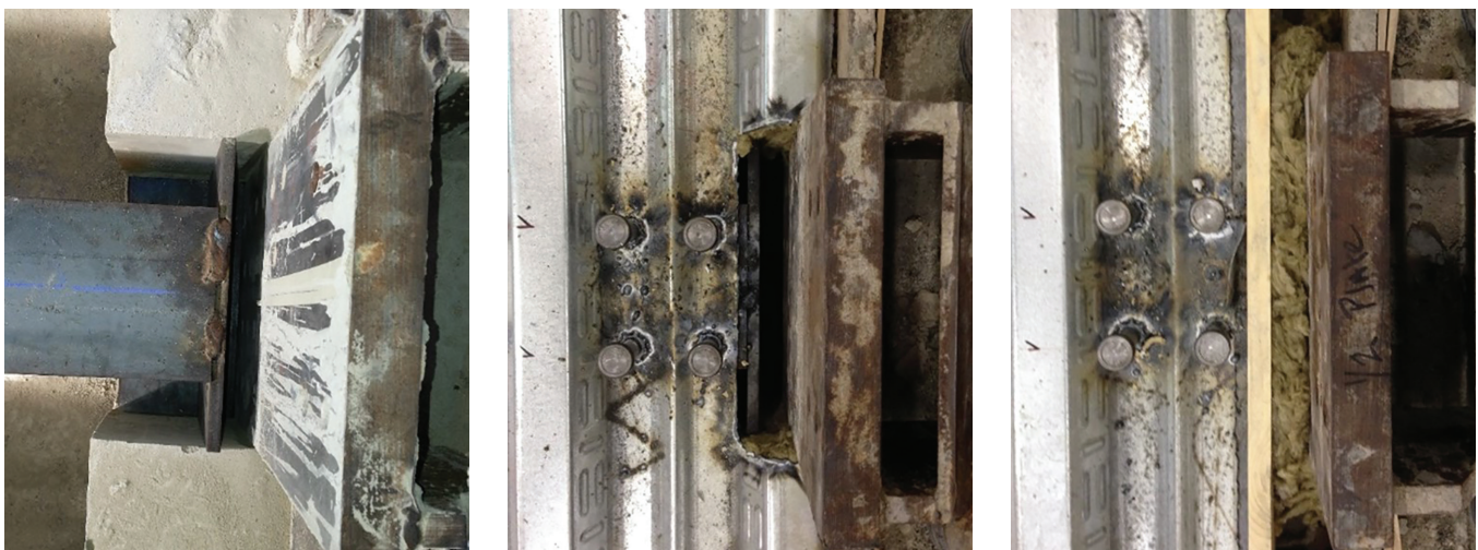
(a) Typical cap-plated beam end prior to deck installation
