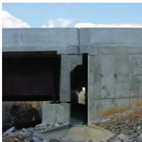
Fig. 11. Virginia Abutment (Hoppe et al., 2016).
