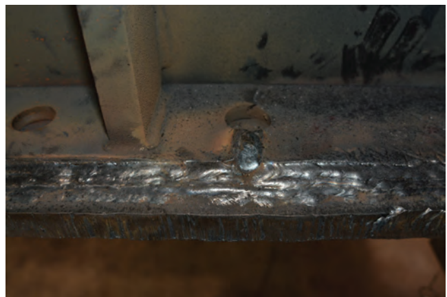
Fig. 9. Bottom flange repair with welded plate of Specimen 4E-1.5-1.75-36a.
