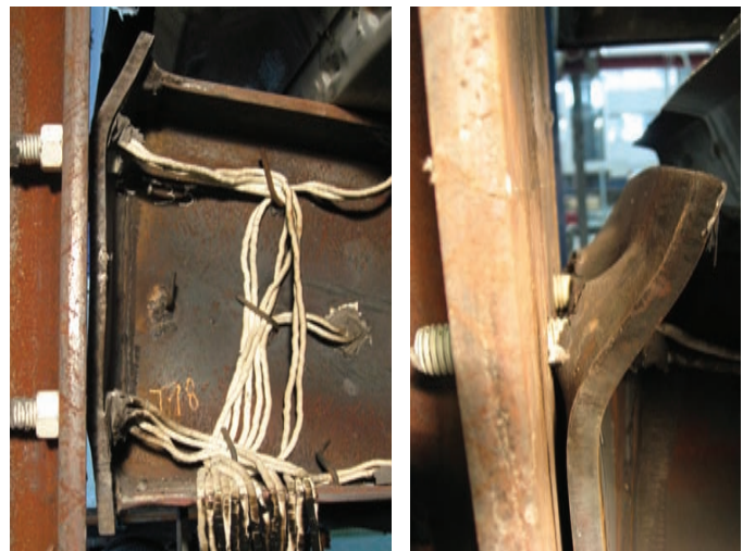
Fig. 16. Joint deformation at test FJ01.
