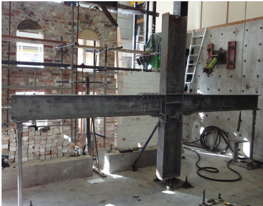
Fig. 10. Full-scale frame subassembly test setup. (Photograph courtesy of Professor G. Charles Clifton)
