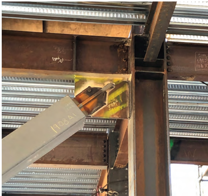
Fig. 5. Traditional gusset at column.
