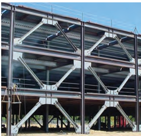
Fig. 2. Typical braced frames with gussets.
