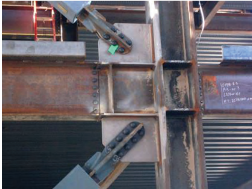
Fig. 4. Full-height gusset brace connection at column.
