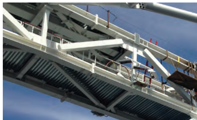
Fig. 3. Truss with gussets.
