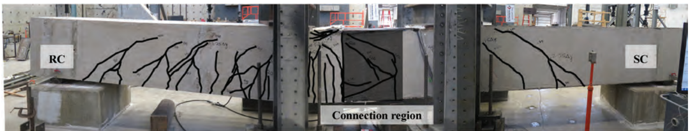
Fig. 21. Concrete crack pattern (east side)—specimen OOPM-C.
