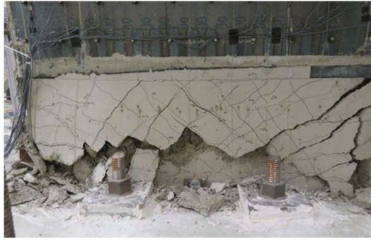
(a) Elevation view RC wall portion
