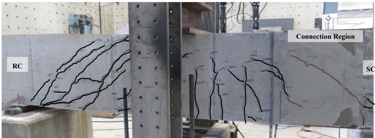
Fig. 29. Concrete crack pattern (east side) (OOPV-DN).
