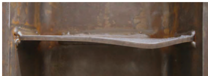
(c) Continuity plate buckling in experiment
