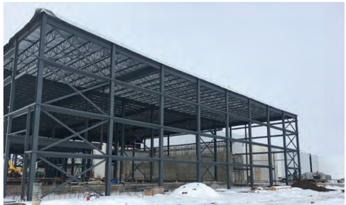
(c) Four-tiered concentrically braced frame
