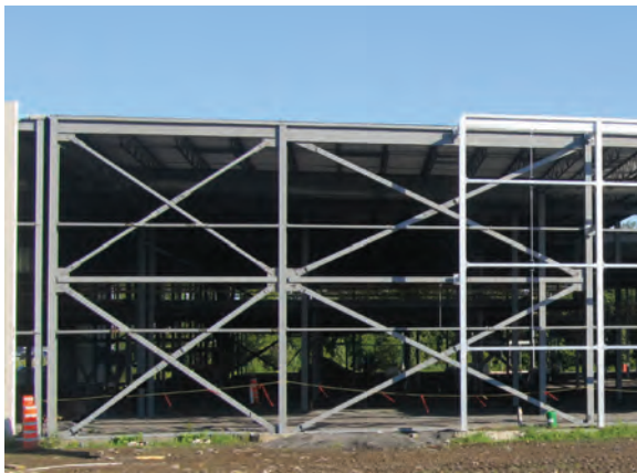
(b) Two-tiered concentrically braced frame
