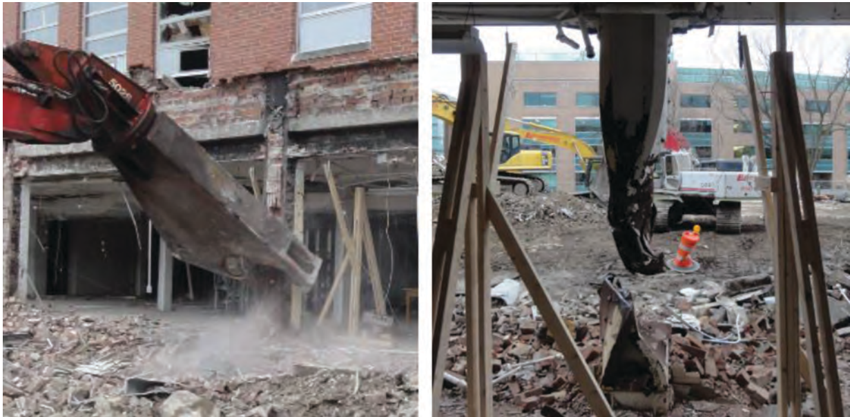
Fig. 7. Column 27 under removal (left) and finished removal (right).
