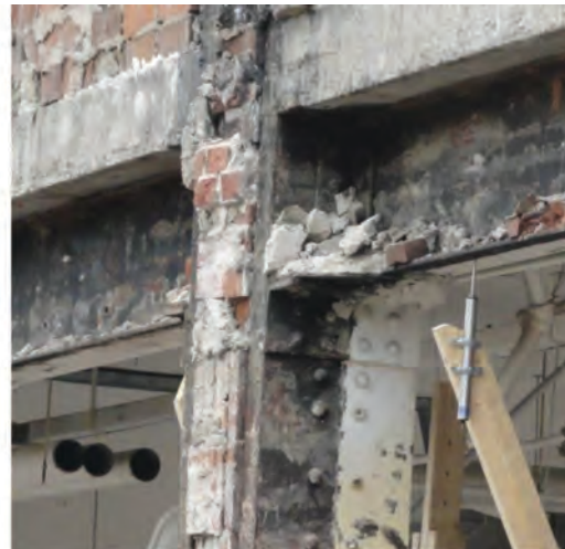
Fig. 4. Close-up detail of column 27 encased in concrete (partial plan view from original drawings), and beam-column connection with rivets through angle on beam bottom flange and web.
