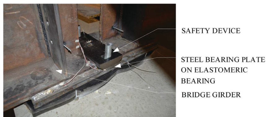
Fig. 12. Safety device at end of physical test.
