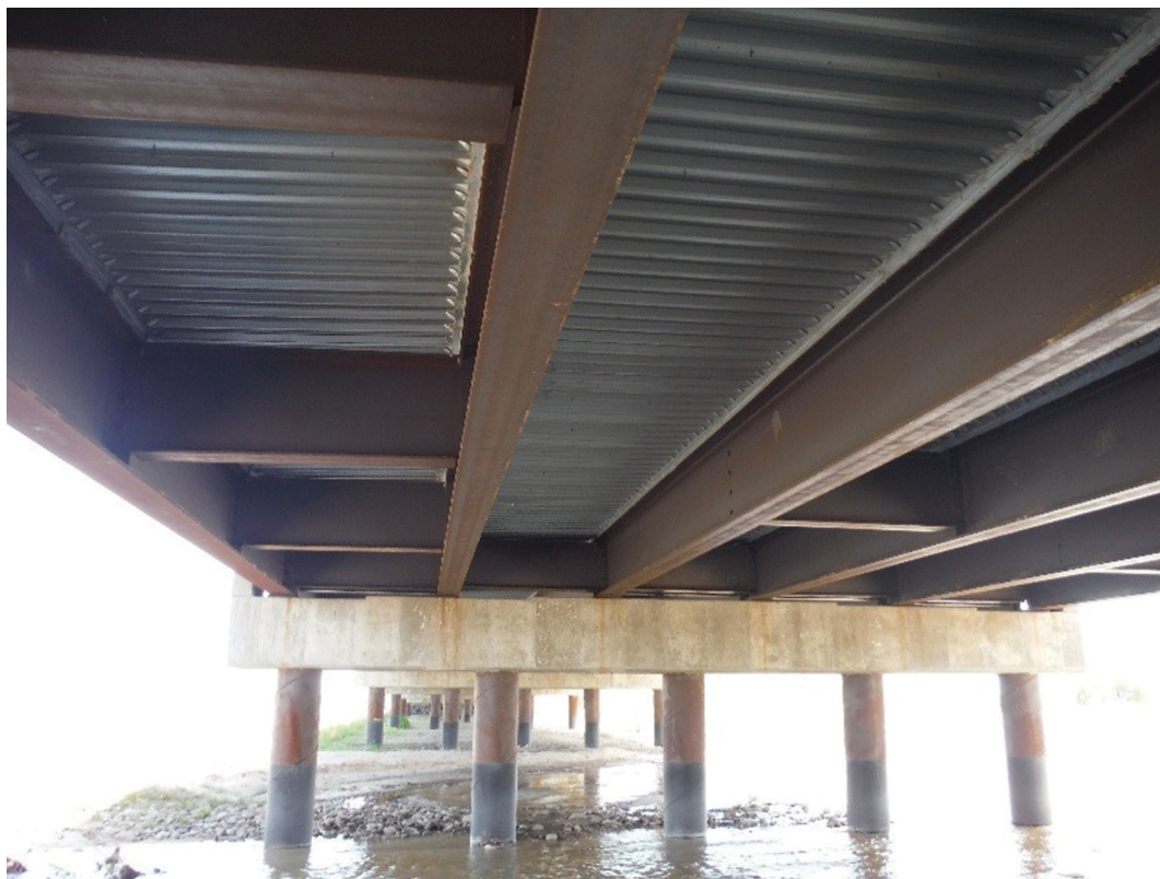
Fig. 2. Bridge over Box Elder Creek, 2015.
