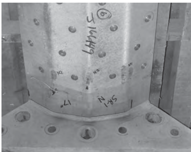
Fig. 13. Specimen SR_1: north crack at upper weld toe after inspection with dye penetrant.
