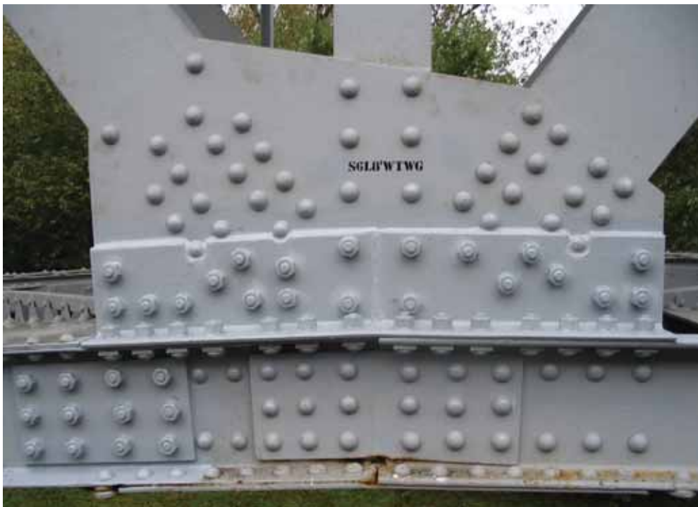
Fig. 11. Efficient repair addressing BCN deterioration.
