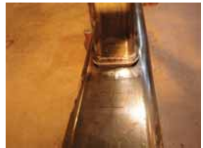
(f) T-0.50-17: chord face rupture
