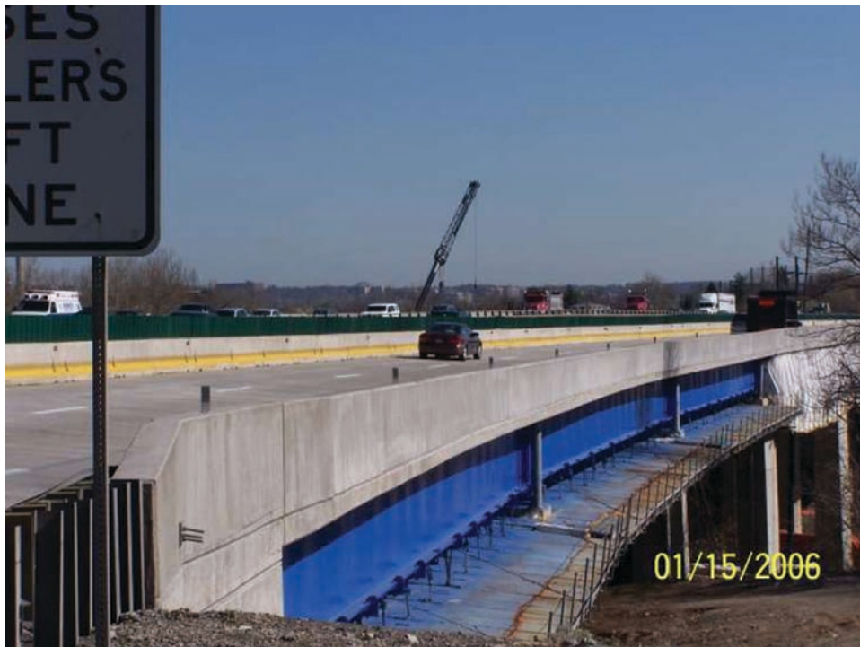
Fig. 12. Reduced number of deck joints.
