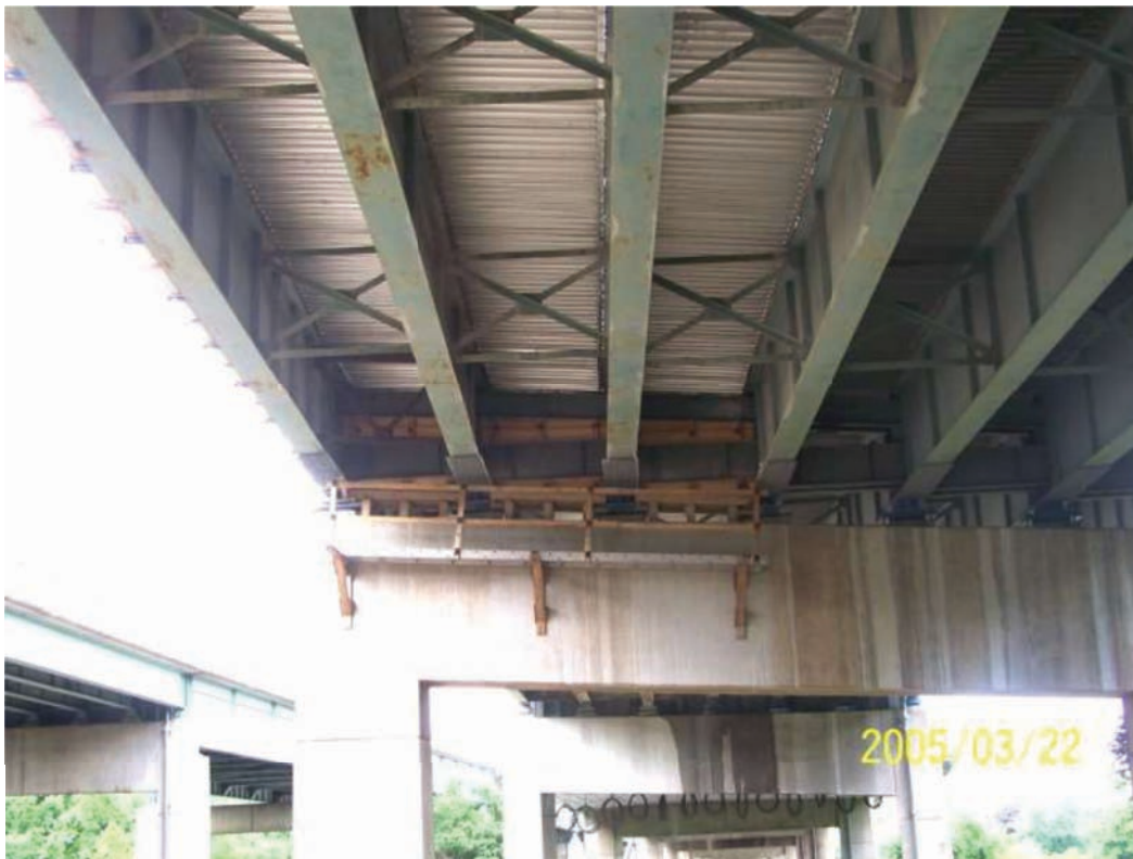
Fig. 5. Formwork for full-depth concrete diaphragm (Section RES construction photo).
