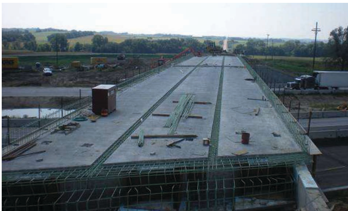
Fig. 25. Before casting the closure regions.
