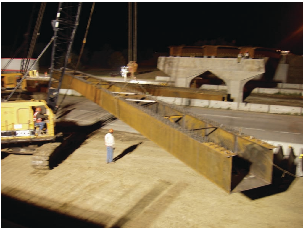
Fig. 6. One of the girders during placement over the support.
