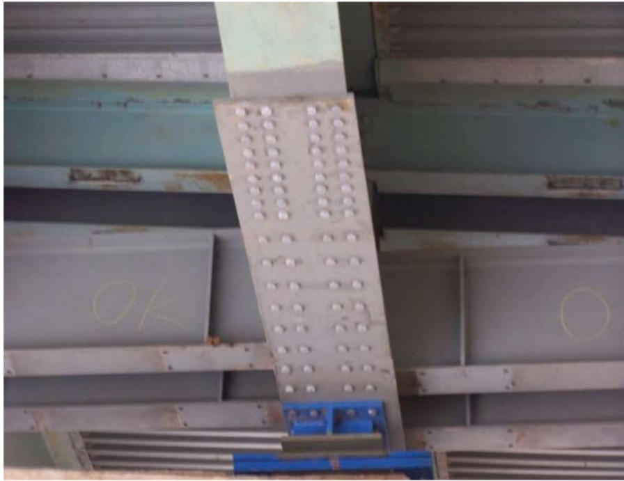
Fig. 6. Bottom-flange cover plate with skewed bolt lines.
