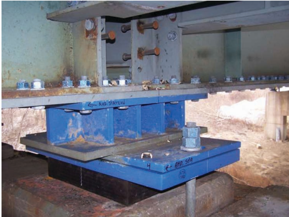
Fig. 9. Elastomeric bearings with steel bolsters.
