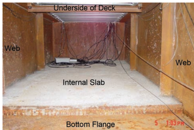
Fig. 5. Inside the box girder near the pier.
