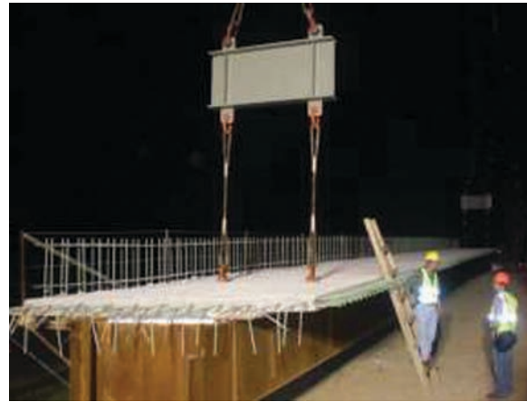
Fig. 21. Lifting of a single pre-topped girder for the 262nd Street Bridge.
