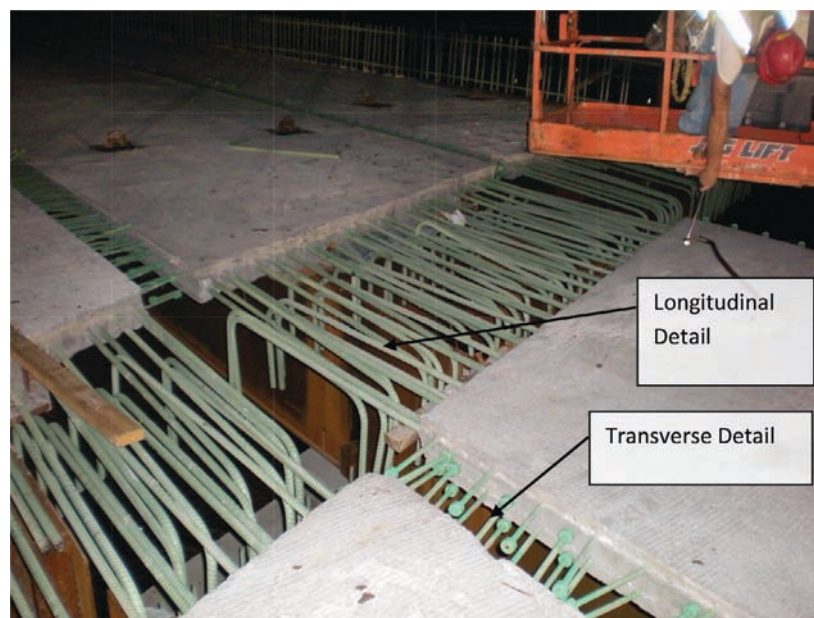
Fig. 19. Accelerated construction closure pier detail.
