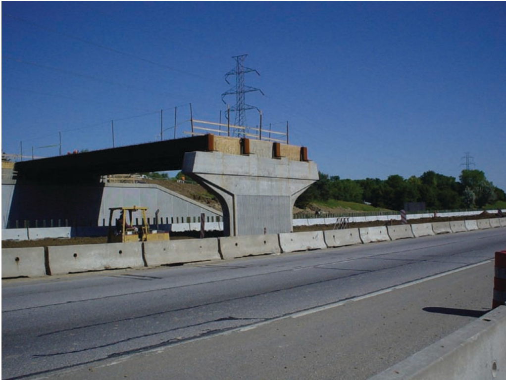
Fig. 14. Erection of first span of Sprague Street bridge over I-680.
