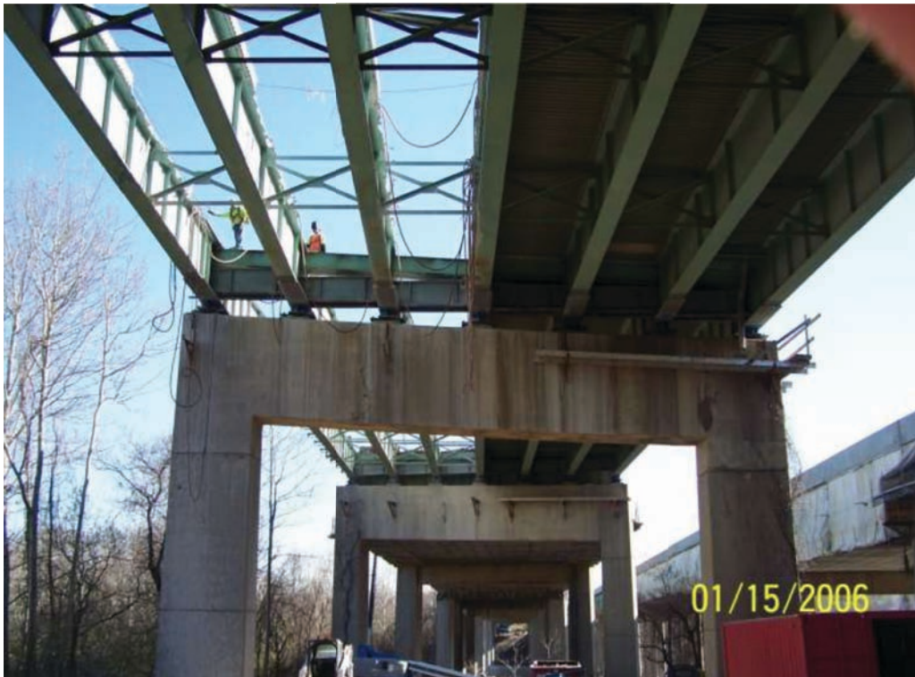
Fig. 2. Approach spans: seven-stringer cross-section during half-width redecking.
