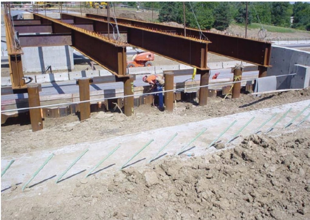
Fig. 15. Erection of first span of Sprague Street bridge over I-680.
