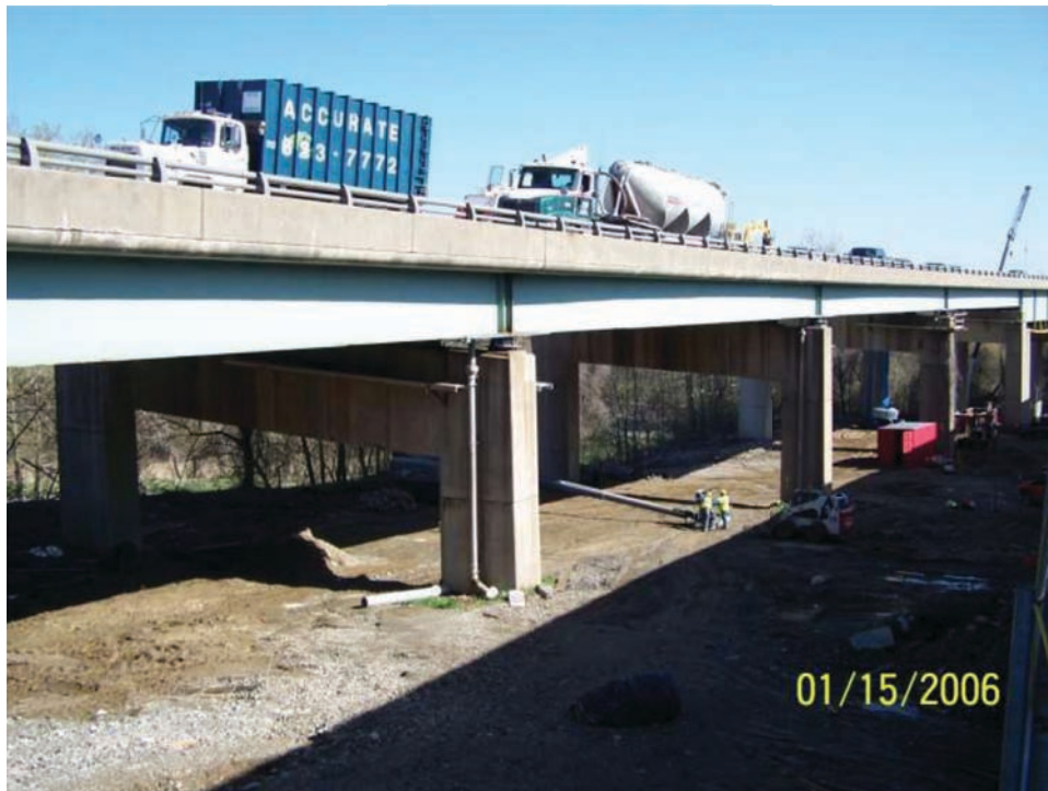
Fig. 3. Southbound approach spans: existing simple-span condition.
