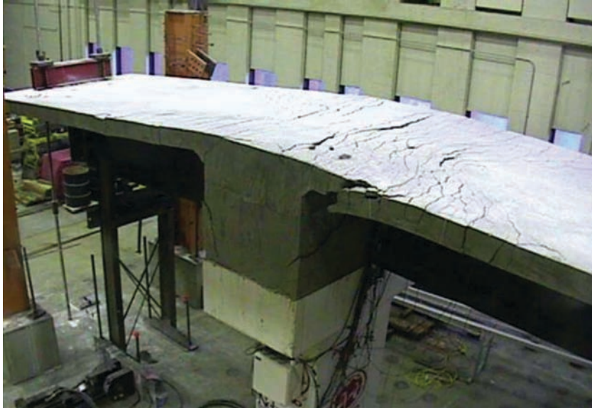
Fig. 17. Photo of specimen after conclusion of test.
