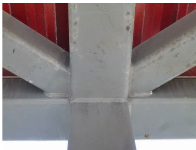
Fig. 1. HSS KT connection.
