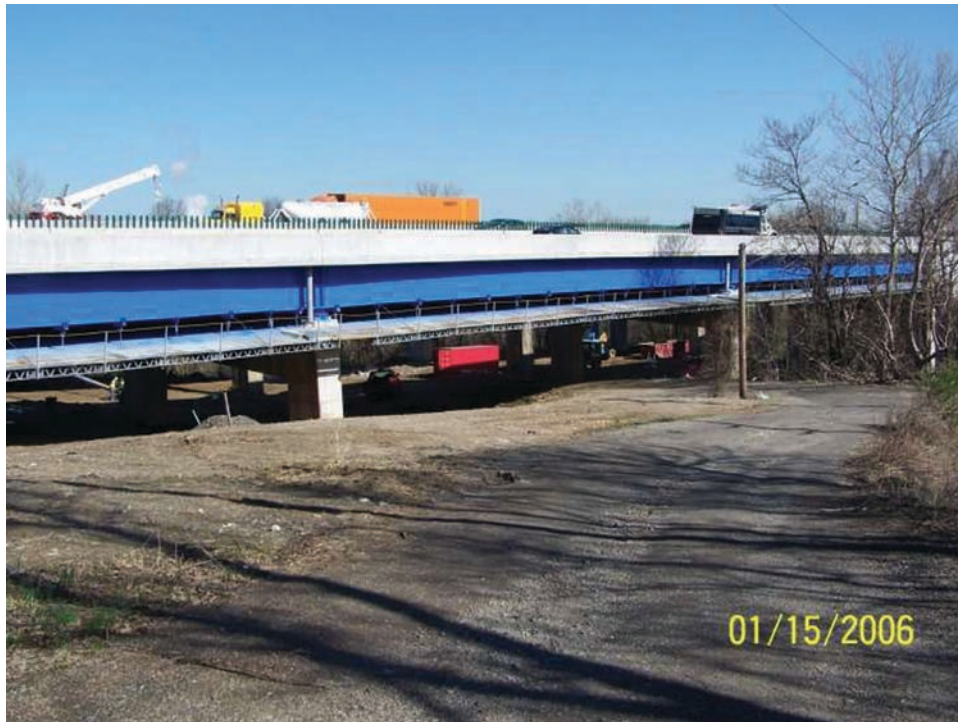
Fig. 11. Completed northbound three-span structure.
