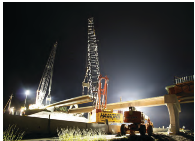
Fig. 17. Pickup and placement of pre-topped units on the supports.
