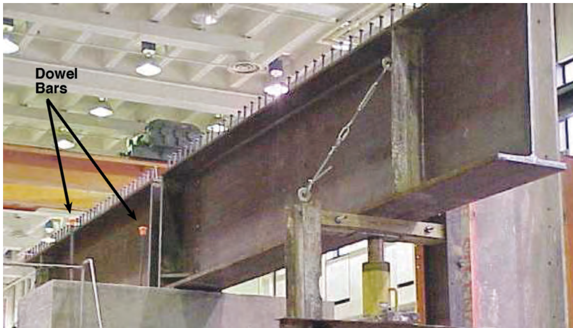
Fig. 5. Photo of the two girders during construction.
