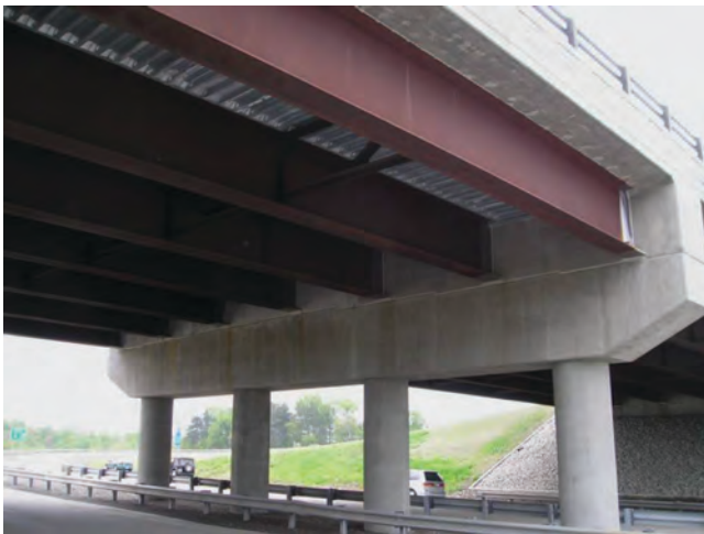
Fig. 7. Completed diaphragm.
