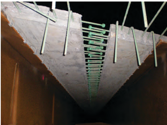
Fig. 20. Possible detail for longitudinal closure pour.
