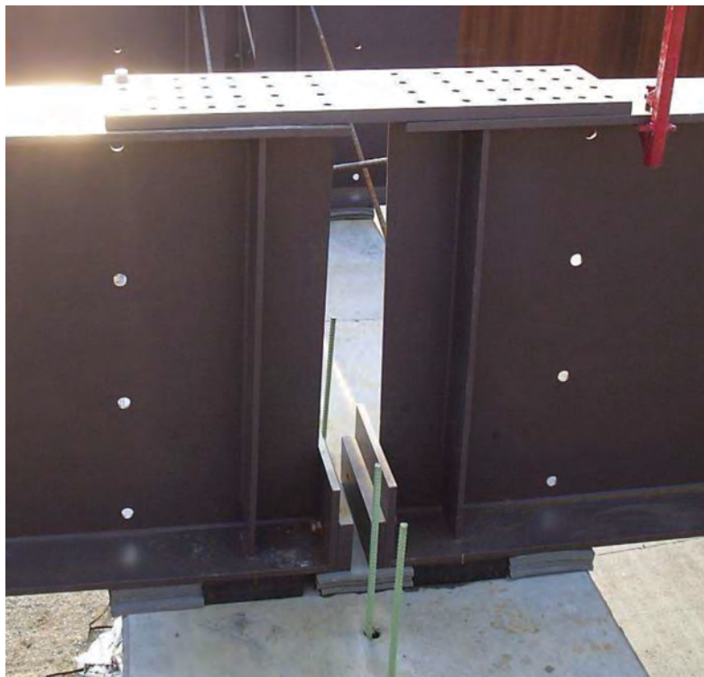
Fig. 6. Three Springs Drive continuity splice.
