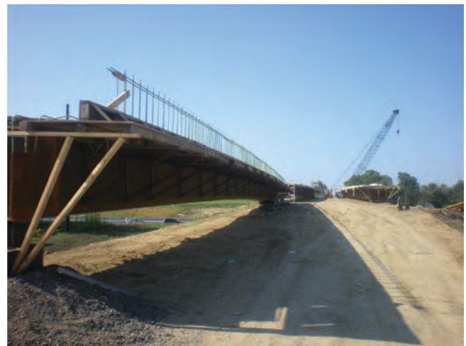
Fig. 16. Preparing the formwork for casting the deck on the unit.
