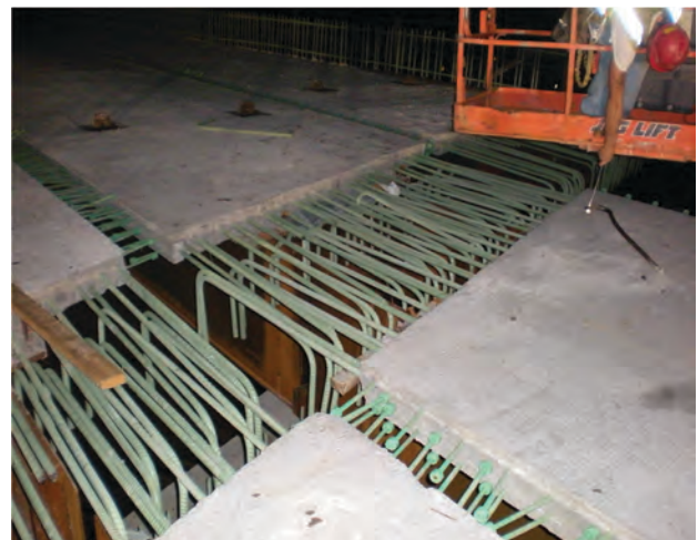
Fig. 19. Recommended interior support detail for an SDCL system used in an ABC application.
