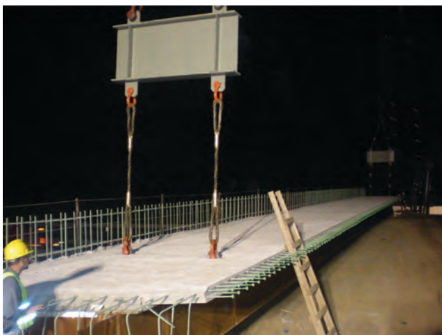
Fig. 17. Pickup and placement of pre-topped units on the supports.
