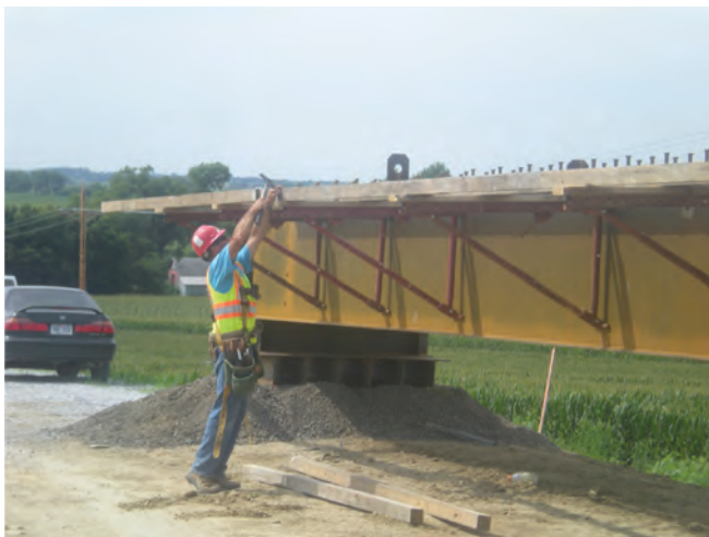
Fig. 16. Preparing the formwork for casting the deck on the unit.
