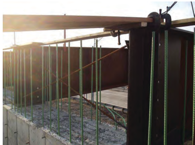
Fig. 8. Temporary cross frames at supports.
