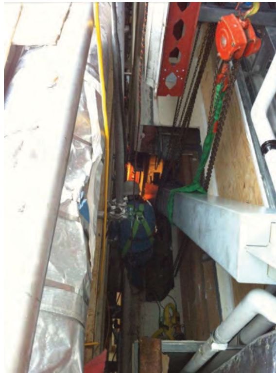
Fig. 27. Spliced BRB installation.
