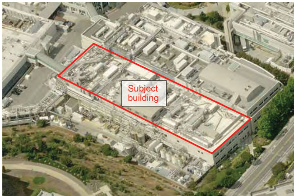
Fig. 1. Aerial view of the facility showing the subject building.
