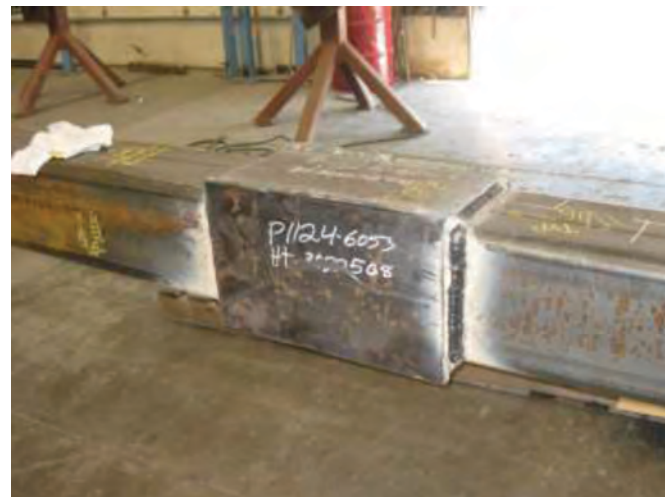
Fig. 10. Finished splice.
