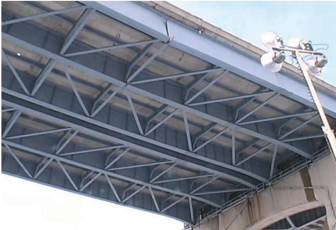
Fig. 11. Two of three girders with full-depth fractures in the Hoan Bridge in Milwaukee, Wisconsin (photograph courtesy of Professor William Wright).
