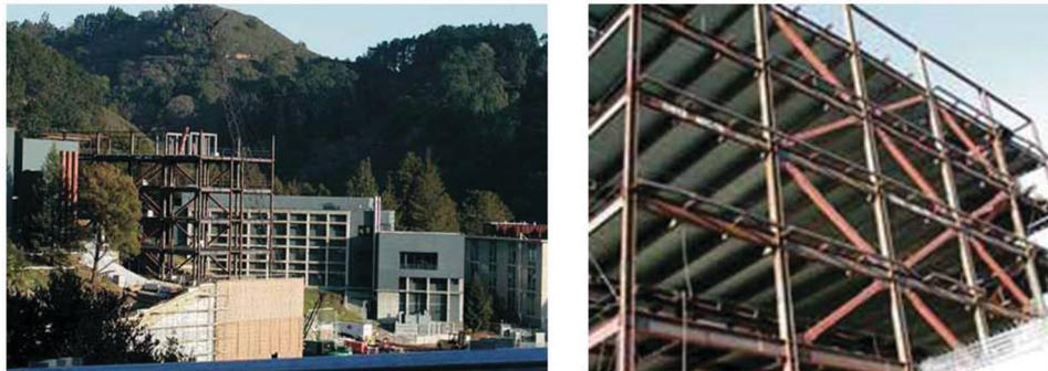
Fig. 1. BRBF Example: Lawrence Berkeley National Lab (Star Seismic).
