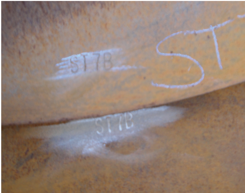
Fig. 1. Example of stamped piece marking at a connection.
