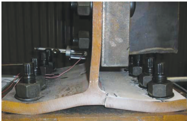
Fig. 13. Example phase 2 flange fracture location.
