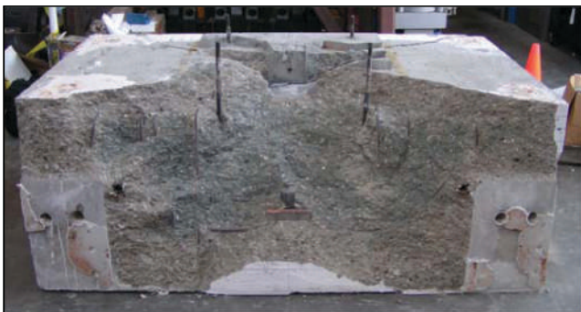
Fig. 14. Edge breakout failure surface of concrete footing (test 6).
