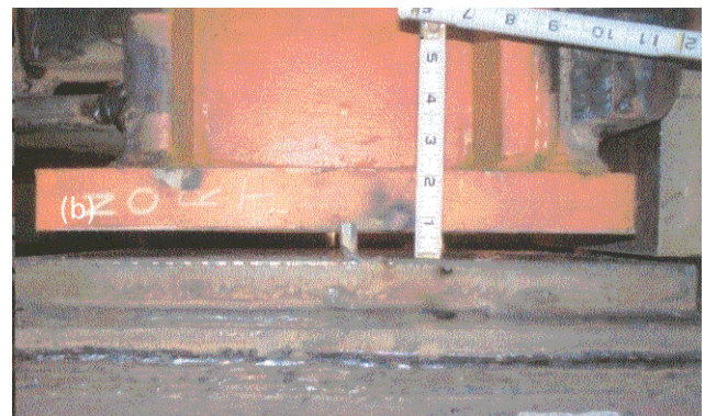
Fig. 8. Rocking displacement at the base of a column of the SC-CBF (Courtesy of Professors James M. Ricles and Richard Sause).
