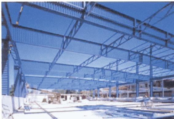
Fig. 2. Storage warehouse with corrugated web girders (Photo courtesy of Professor Hartmut Pasternak).
