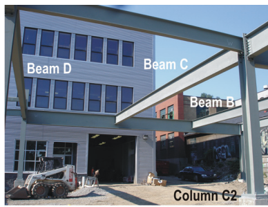
(a) Beams B, C and D during erection.
