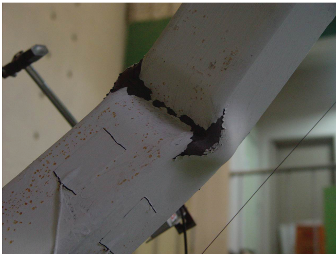
Fig. 4. Local buckling of brace 100×100×6.
