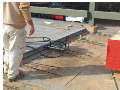
(e) Pulling PT strand near beam A.
