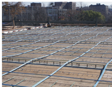
(b) Deck prior to concrete placement.
