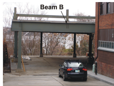
(g) Completed structure looking East showing beams A and B.
