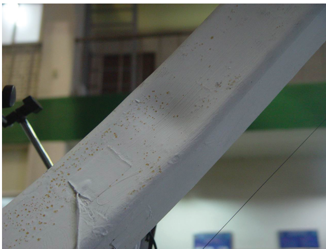
(c) Local buckling (-2%).
