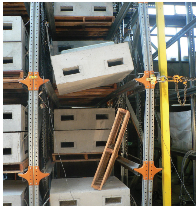
Fig. 7. Pallet-loading-induced failure of storage rack (notice the damaged upright on the right-hand side of the photograph) (Photo courtesy of Professor Kim Rasmussen).
