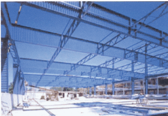
Fig. 2. Storage warehouse with corrugated web girders (Photo courtesy of Professor Hartmut Pasternak).
