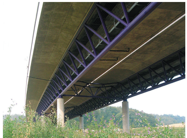
Fig. 1. Bridge with tubular truss beams.
