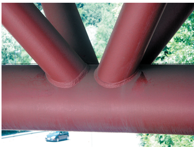
Fig. 2. Truss connection with circular hollow structural sections.
