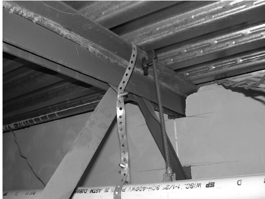
Fig. 7. Joist with crimped web members.
