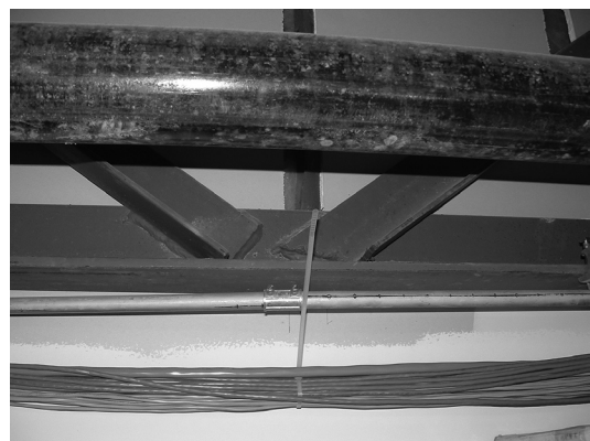
Fig. 14. Web angles on side of chords.
