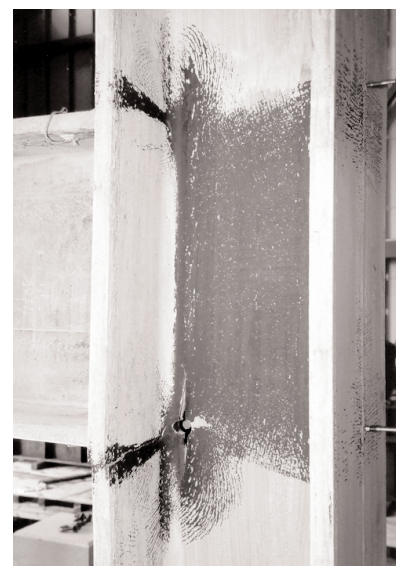
(b) Column Flange Fracture
