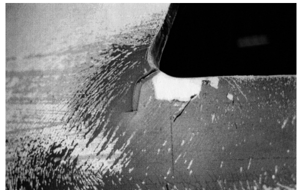
Fig. 14. Crack at opening corner (Specimen B2).
