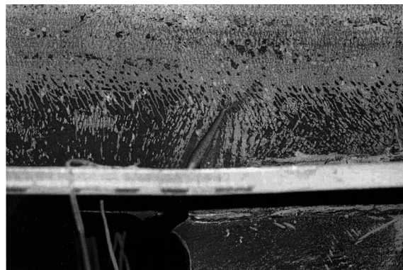
Fig. 18. Crack at opening corner (Specimen B4).
