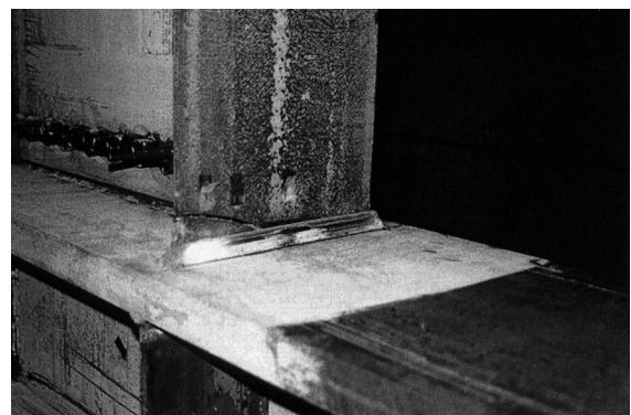
Fig. 12. Fracture of bottom flange (Specimen B1).
