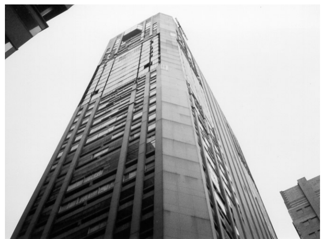
Fig. 1. High-rise steel framed building showing boarded up floors near the top where a fire occurred.
