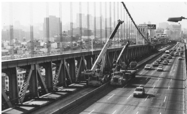
Fig. 6. Benjamin Franklin Bridge - placement of new deck panels in exterior lane.
