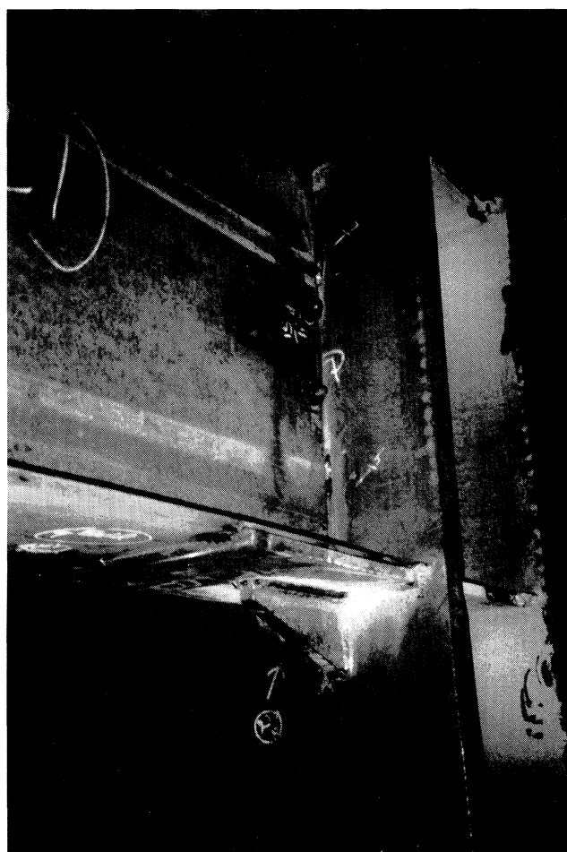
Fig. 6. Specimen ready for field welding: side opposite the shear tab.
