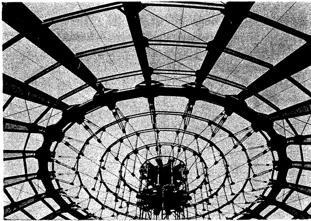
Fig. 19. View of cable roof, Travelers Insurance Pavilion
