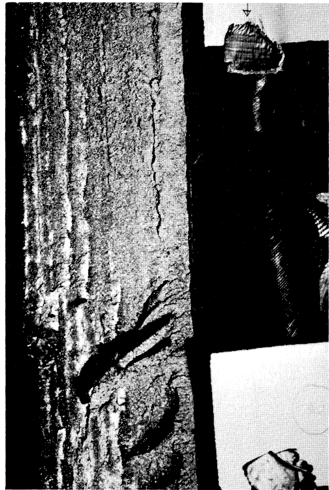
Fig. 10. Failure surface of partial penetration welded splice—center of bottom flange.
