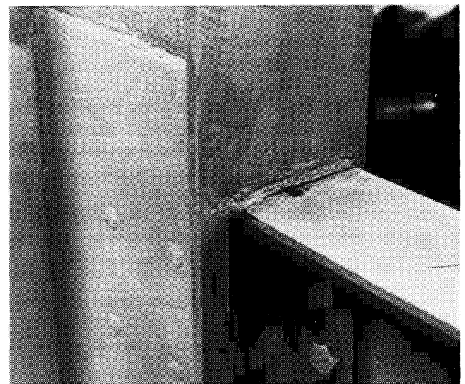
Fig. 10. Specimen 1a instrumentation arrangement and 1b failure location
