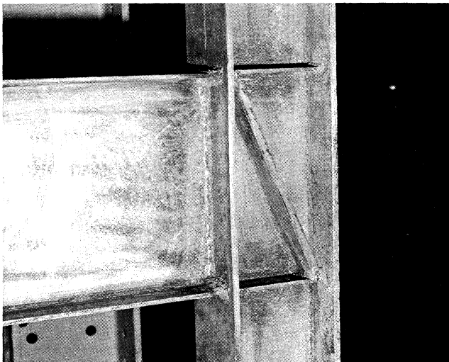
Fig. 5. Exterior beam-to-column connection
