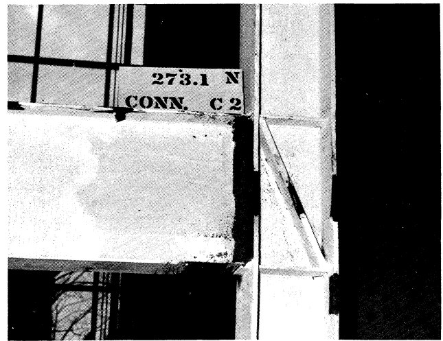
Fig. 23. Exterior connection, diagonal stiffener in tension
