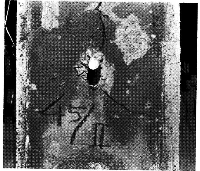
Fig. 4. Grout failure; load applied at 45°
