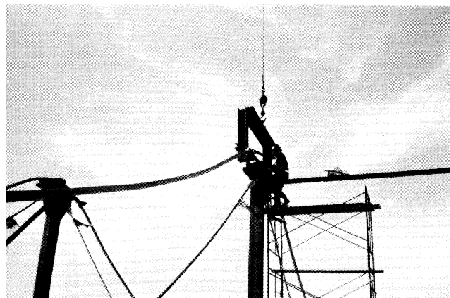
Fig. 4. Placing the outer cable atop the mast using the lifting saddle
