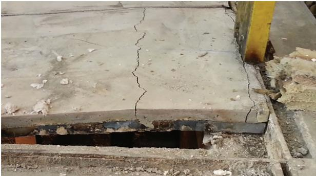
(b) R-C slab edge transverse cracking
