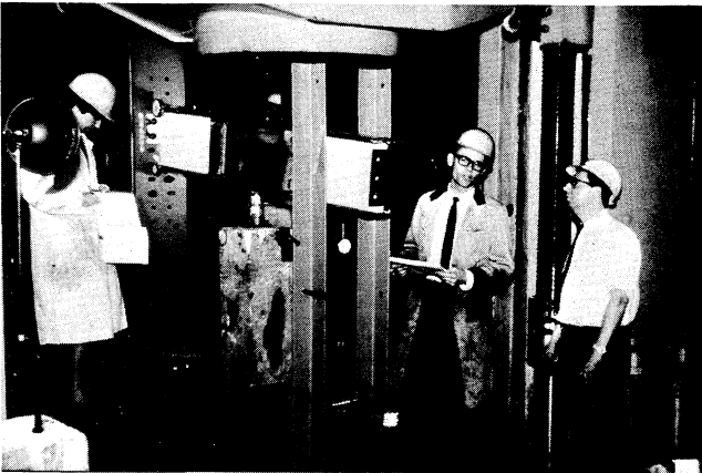
Fig. 3. End plate test jig and specimen
