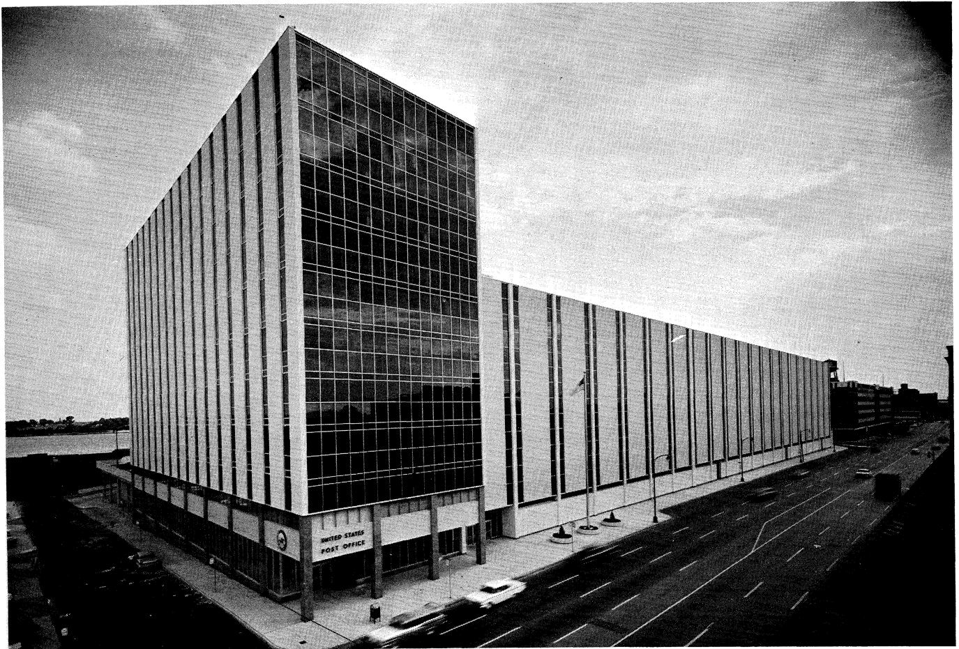
Fig. 2. Detroit U. S. Post Office, view looking west; Fort Street elevation.
