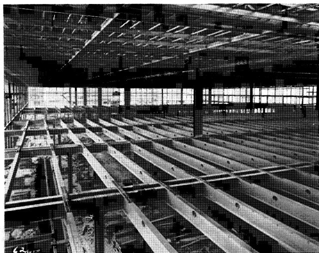
Fig. 7. Steel framing, Hall C, view looking north. Note 60 ft span beams framing into double girders.
