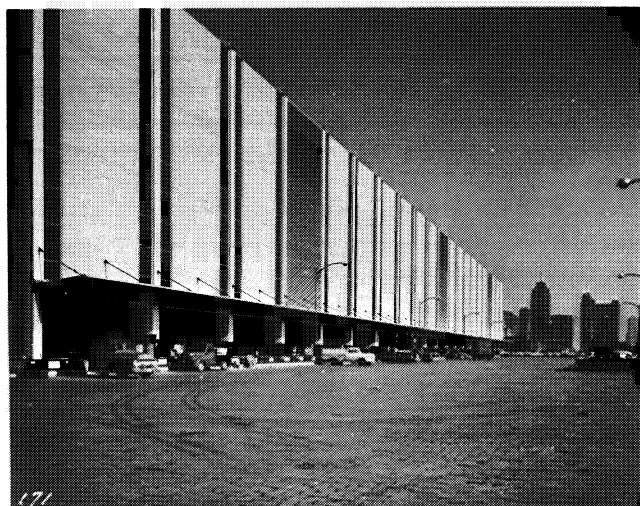
Fig. 14. U. S. Post Office, south maneuvering area, view looking east.
