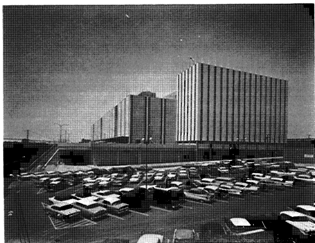
Fig. 11. U. S. Post Office, view looking west. South maneuvering area on the left.
