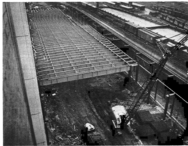
Fig. 12. U. S. Post Office, south maneuvering area, erection of welded plate girders. Note shear connectors shop welded on top flange.
