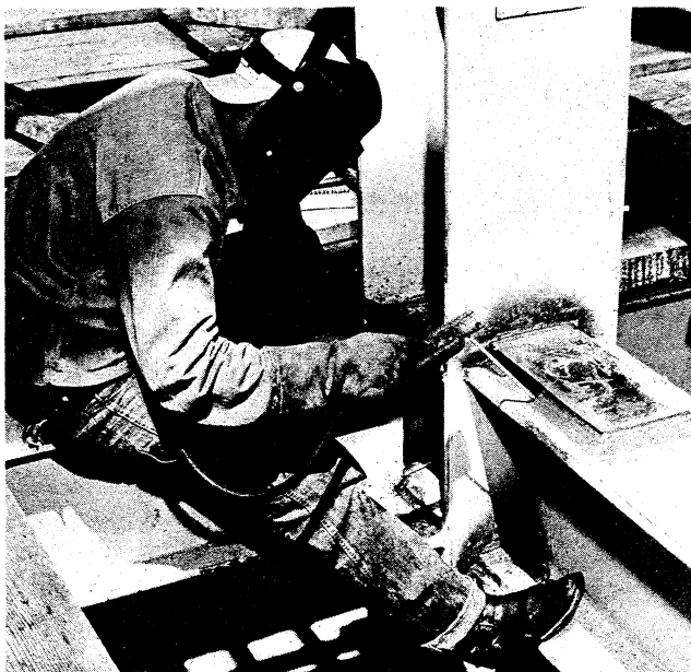
Fig. 2. Welded moment connection
