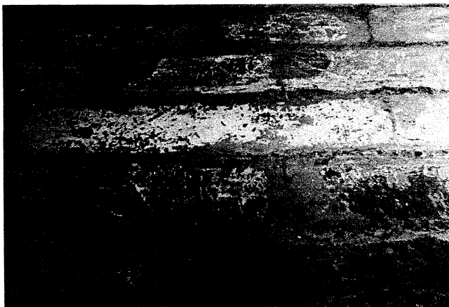
Fig. 5. View of typical deck surface condition, revealing only shallow corrosion marks and pits. Corresponding profile is shown in Fig. 7b
