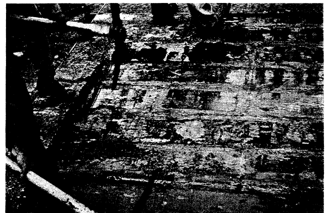
Fig. 3. Removal of planks by pick. Shiny surfaces are areas where the bond between the plank and the deck was intact
