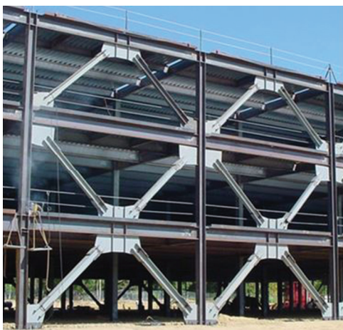
Fig. 2. Typical braced frames with gussets.
