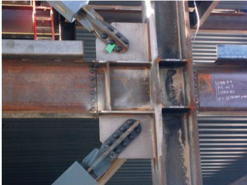
Fig. 4. Full-height gusset brace connection at column.
