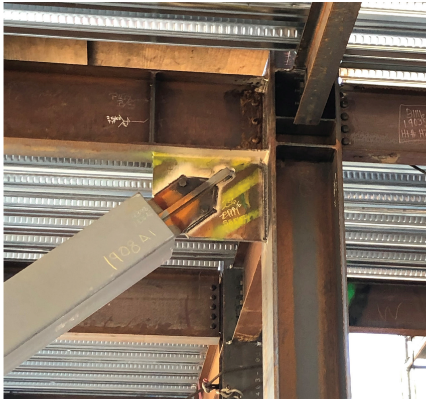
Fig. 5. Traditional gusset at column.
