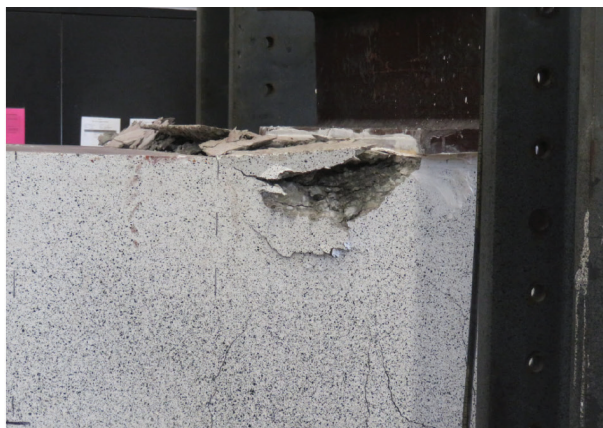
(a) Concrete crushing at the RC loading point
