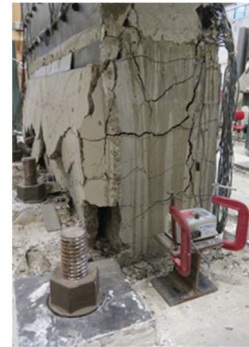
(b) Side view RC wall portion
