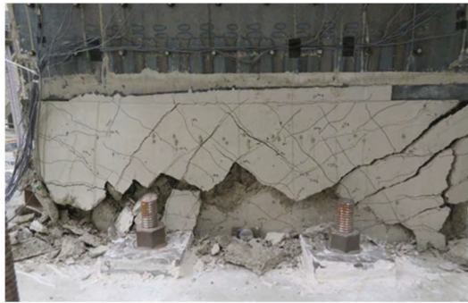
(a) Elevation view RC wall portion
