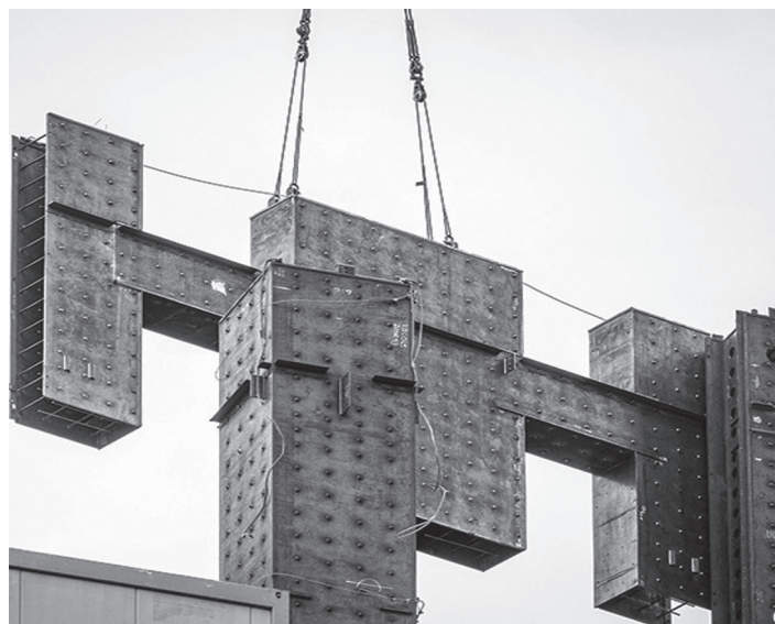
Fig. 2. Assembled coupled C-PSW/CF module being lifted into place at Rainier Square Project in Seattle, Washington (photo courtesy of Keith Evans/ENR).
