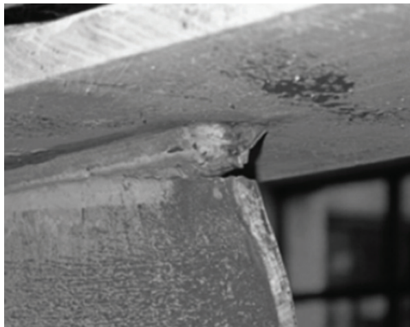
(a) During the test
