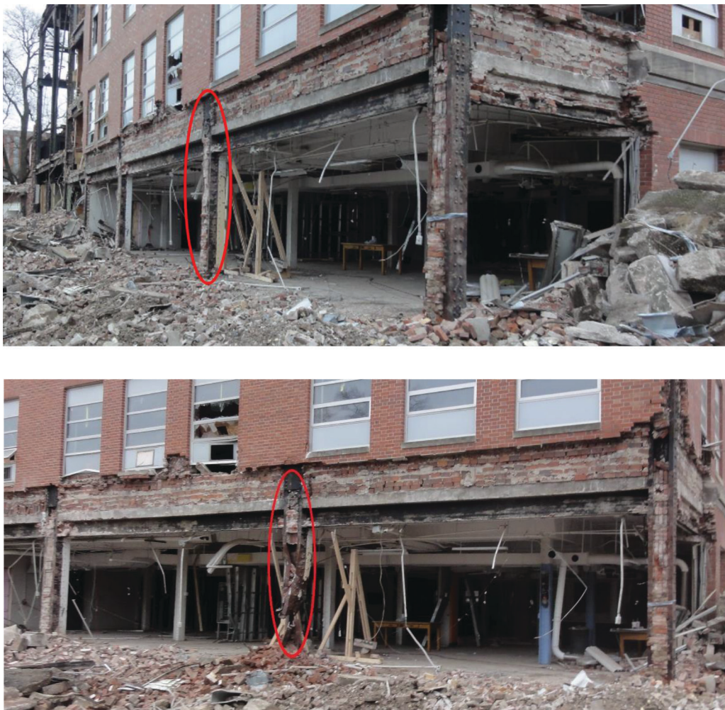
Fig. 8. Penultimate column 27 before removal (top) and after removal (bottom).
