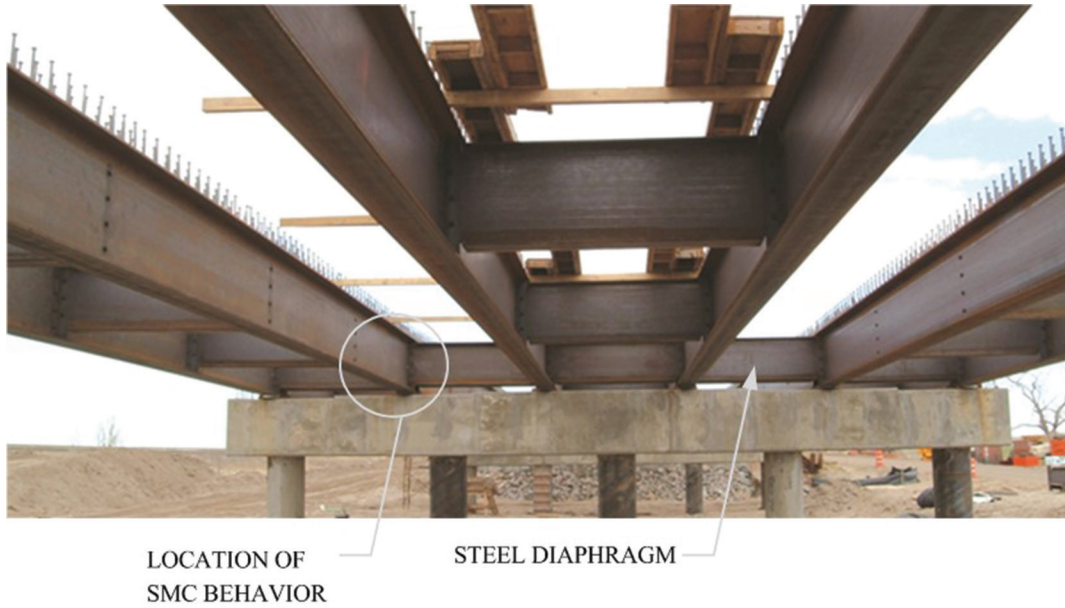
Fig. 1. Bridge over Box Elder Creek, 2005 (reprinted courtesy of AISC).
